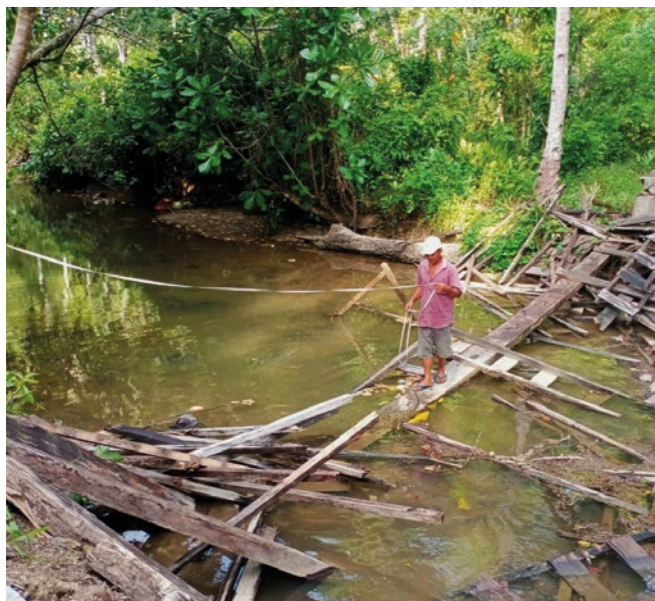
Collapsed bridge on the way to the nesting beach
